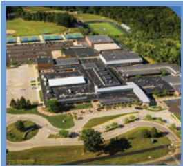
Learning environments, roofing, mechanical, paving
