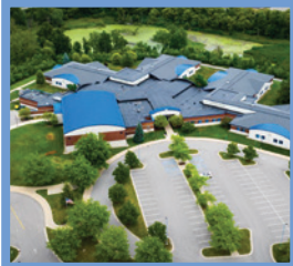
Learning environments, mechanical, paving, playground
