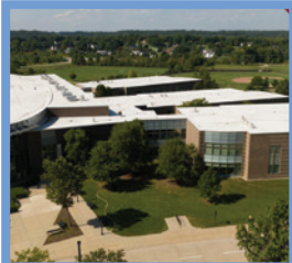
Mechanical, paving, roofing, additional access drive
